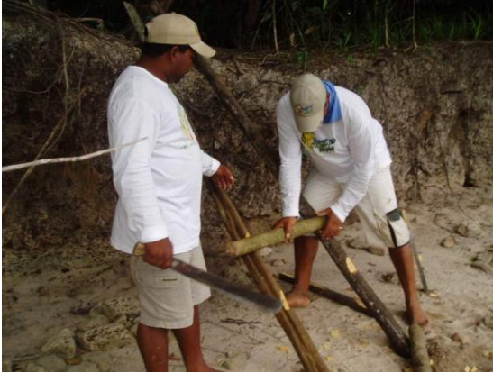
Building the Ladder
